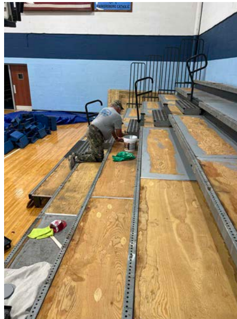
Ed Franks “cutting in” around the stairs.
